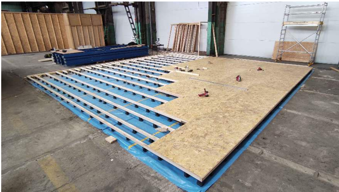
Figure 7.1: Picture of the unfinished wooden floor in Refshaløen
