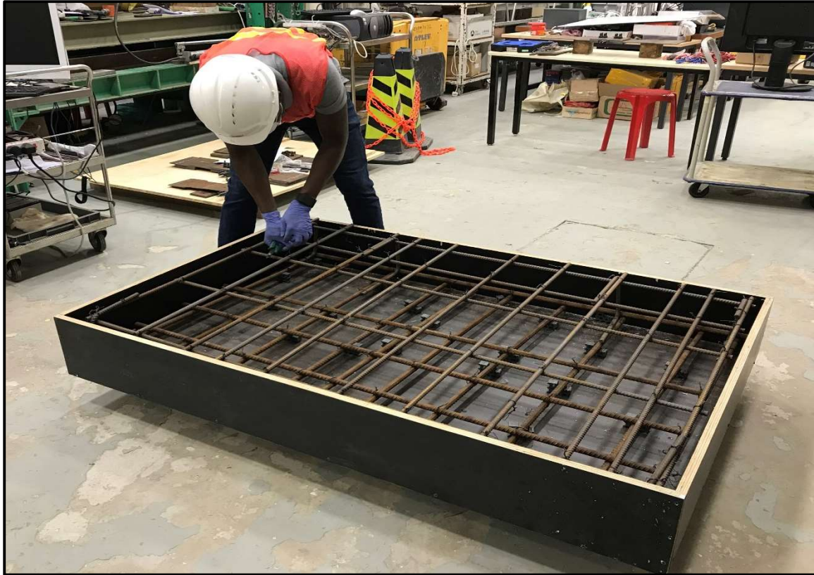
Fig. 3. A simulated manual rebar tying activity
